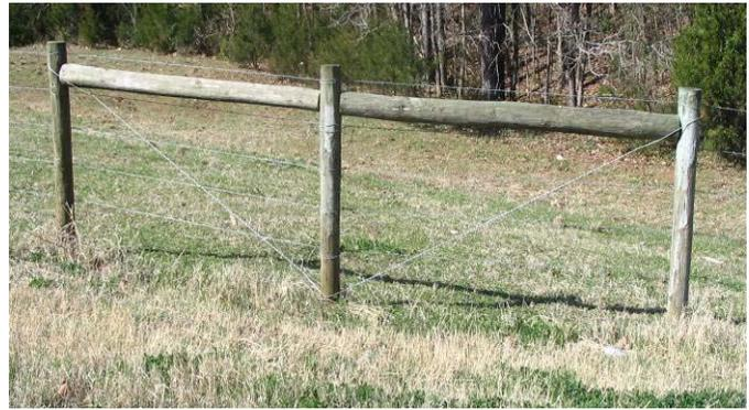
An H-brace is required for all barbed wire fences and electric fences with more than two wires. Since barbed wire fences need to be tight to be effective, a well-built H-brace is very important. This is in contrast to electric fence where the control is by animal fear of the electric fence and the fact that high tensile wire, especially single strand, should not be very tight.
